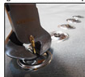
Cut off excess nail shank
