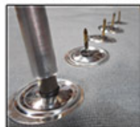
Using the tool, push fastener down onto nail shank
