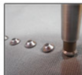
Repeat fastener installation on all cut nail shanks
