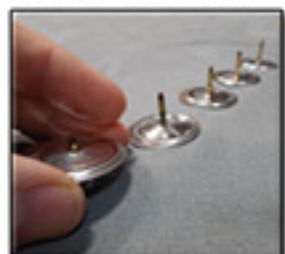
Insert NW1 washer onto nail shank
